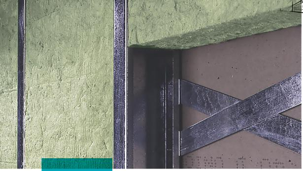
ROCKWOOL AFB<sup>®</sup> is a lightweight, acoustical fire batt stone wool insulation specifically designed for steel stud interior wall and floor applications. Its superior sound absorbency and fire protection contribute to the overall comfort and safety of occupants.
